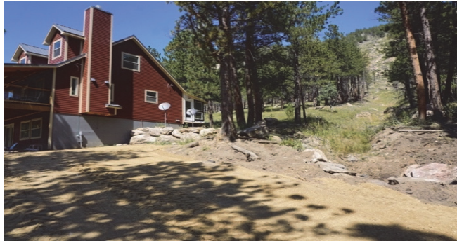
FIGURE 4 NEW HOUSE CONSTRUCTED WITHIN TEN FEET OF THE 2013 DEBRIS TRACK
